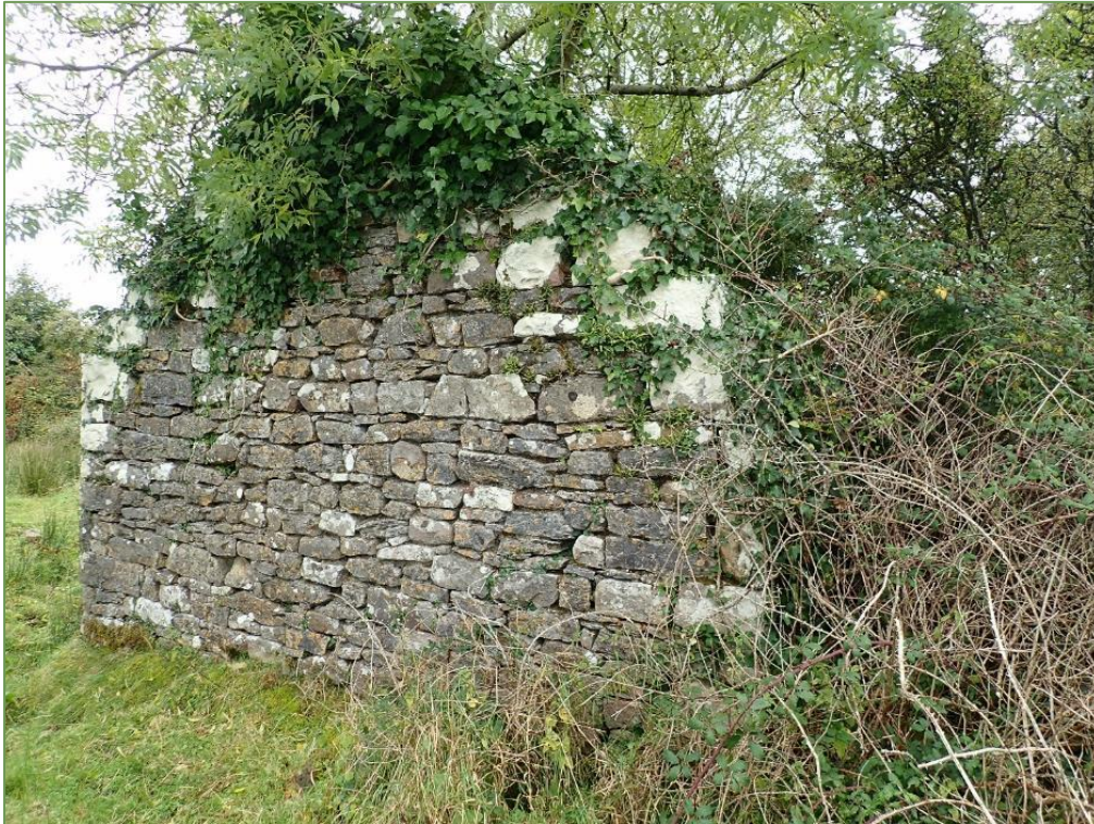
Plate 3.3 - Ruin building adjoining eastern half of site.
